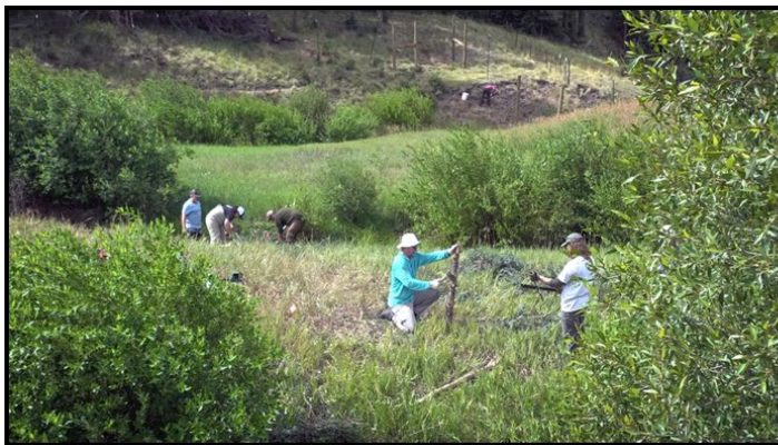
Large woody debris structures on Lagunitas Creek. The structures, combined with channel shaping and point bar above work to stabilize eroding banks, dramatically increasing pool depth and habitat in the reach.
