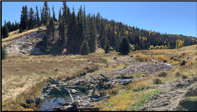
Large woody debris structures on Lagunitas Creek. The structures, combined with channel shaping and point bar above work to stabilize eroding banks, dramatically increasing pool depth and habitat in the reach.
