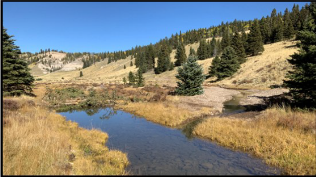
Constructed log jam on the Rio San Antonio splitting the river's flow between current channel and abandoned side channel, providing increased sinuosity and floodplain connectivity Photos by Craig Sponholz
